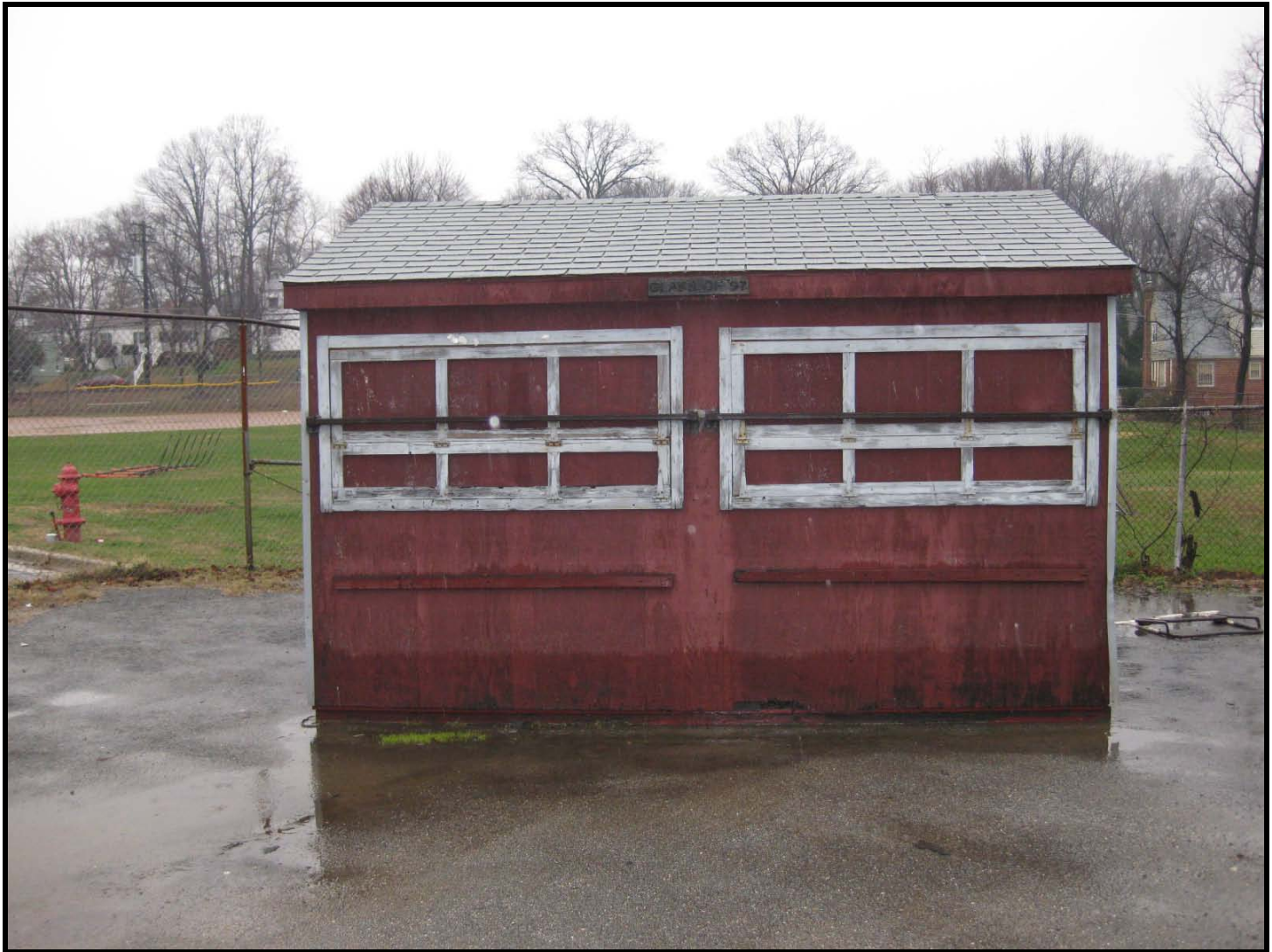
Photo: Ticket Booth, Capitol Heights, façade (southeast elevation), looking northwest. (December 2009)
