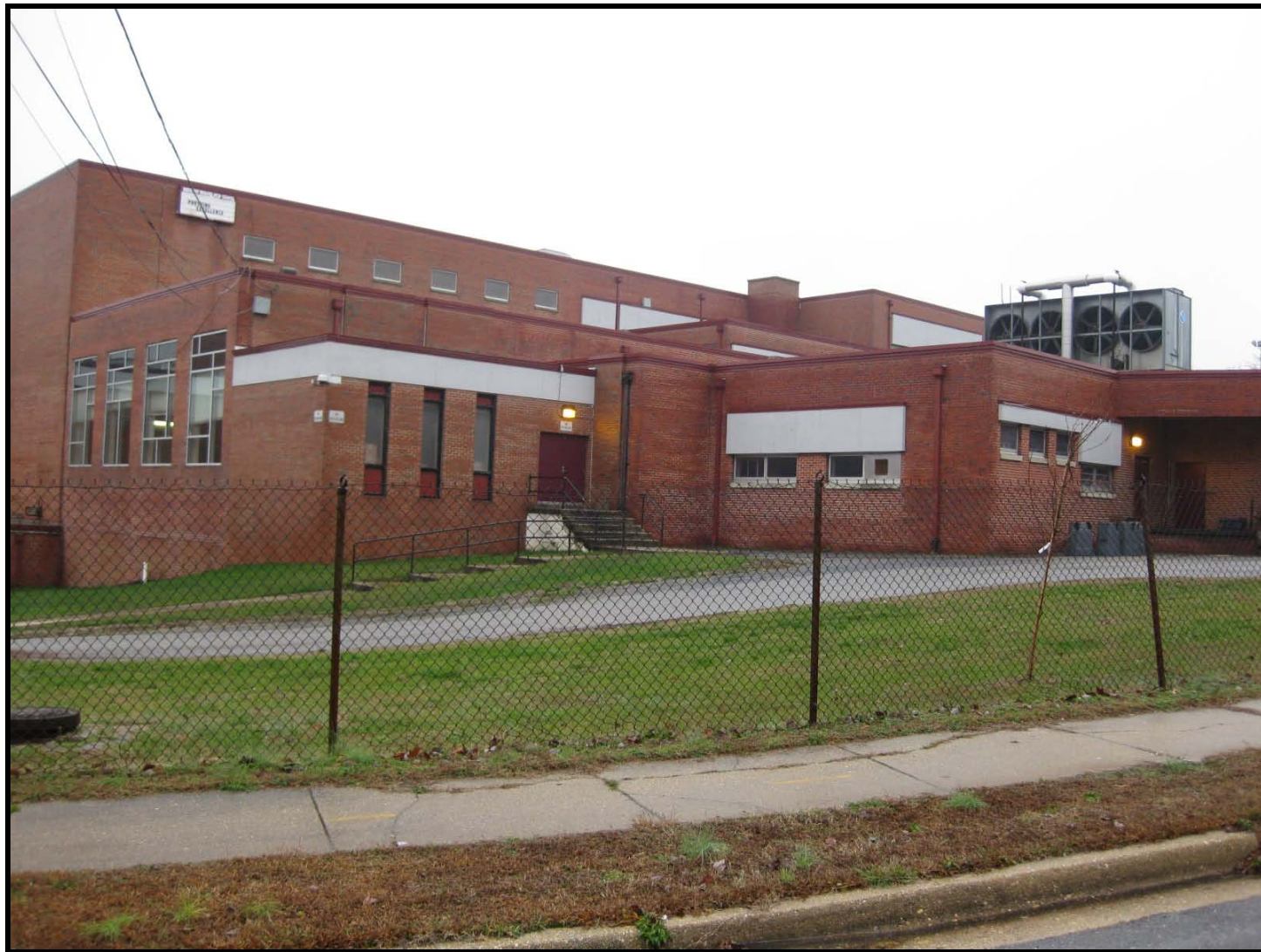
Photo: Fairmont Heights High School, Capitol Heights, view of the western corner, looking east. (December 2009)
